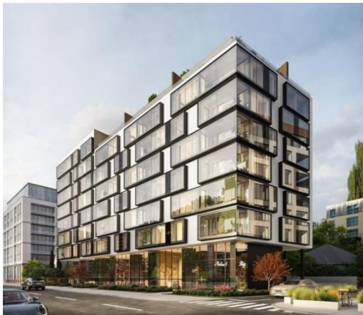
Stambeno-poslovni objekat, ul. Cara Dušana, Niš Residential and office building, Cara Dušana st., Niš
